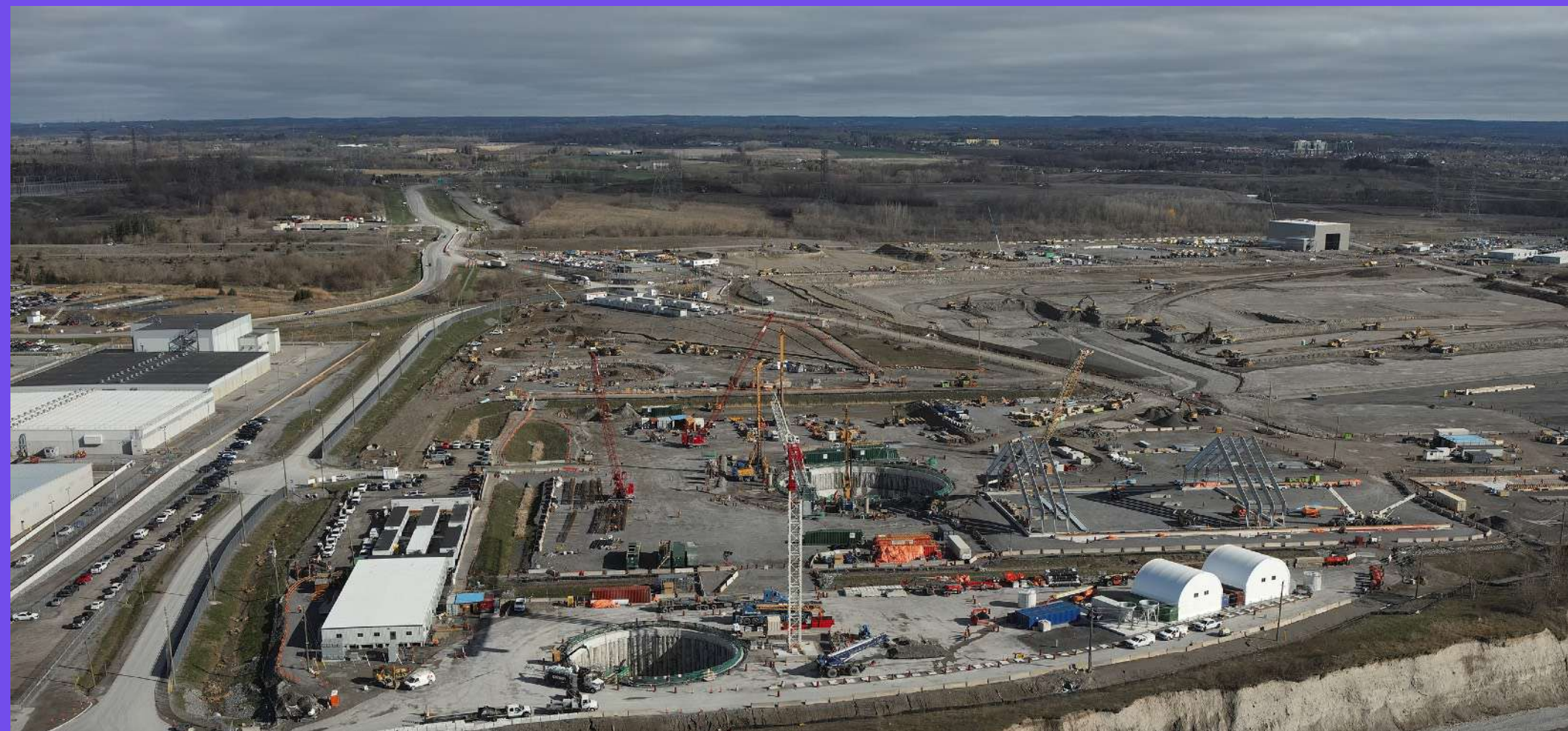
Construction of OPG's first of four BWRX300 SMRs at the Darlington, Ontario site. Source https://www.opg.com/wp-content/uploads/2025/05/DJI_20250430085020_0002_2732_crop.jpg
