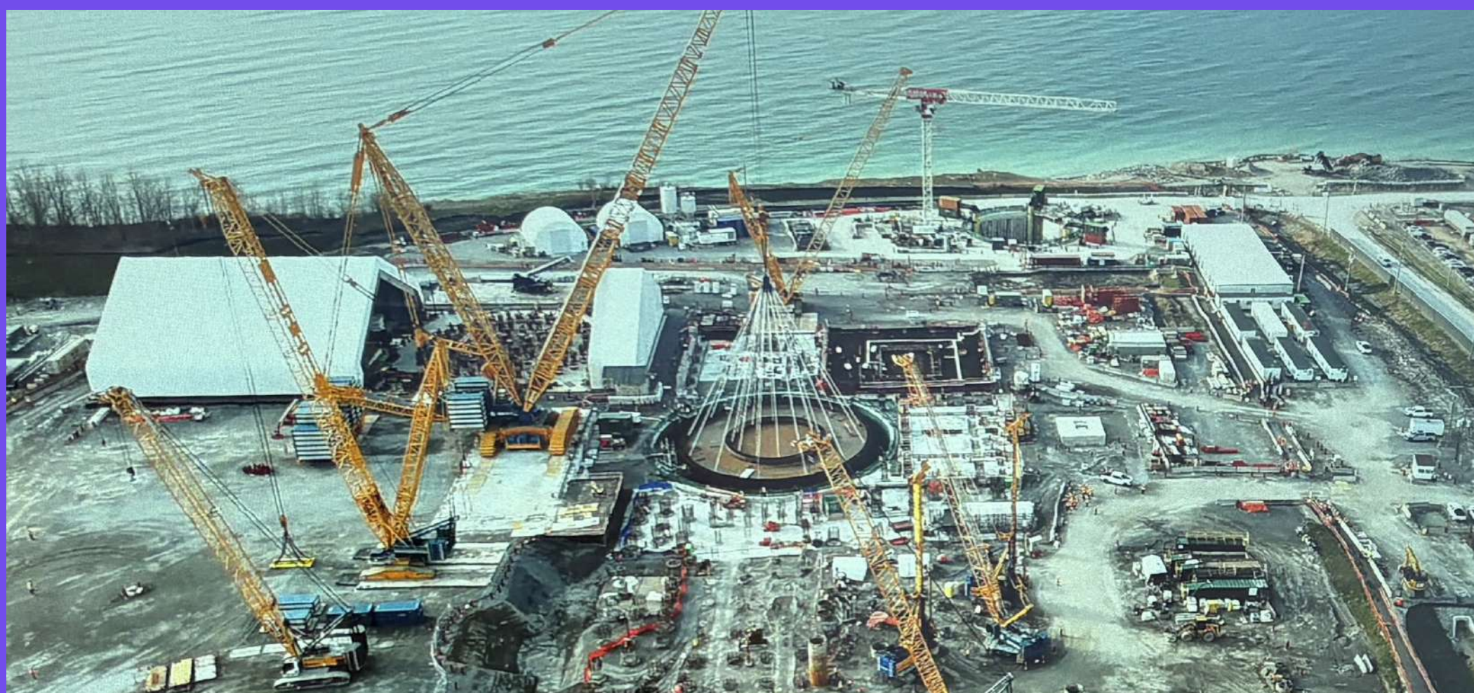
Construction of OPG's first of four BWRX300 SMRs at the Darlington, Ontario site. Basemat foundation being lowered into the reactor shaft. Source https://www.opg.com/wp-content/uploads/2026/04/basemat-lift-april22.png
